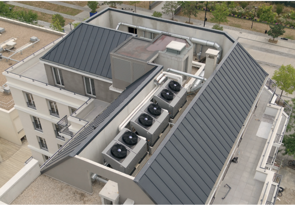
Cascade installation of 80 kW HRC dual-service heat pumps. @ Groupe Intuis.
